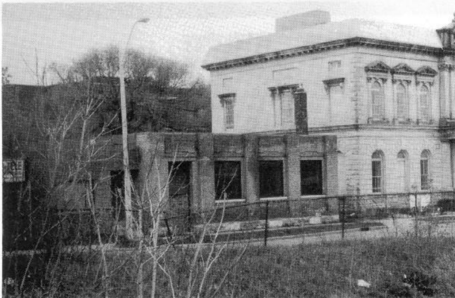
The remains of 41 Stuart Street after the upper floors were destroyed in a 1948 fire. (Williamson)
