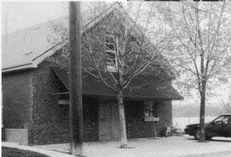
Built in 1869, 469 Bay Street has been designated a historic property and returned to its original use as a sail loft. (R. Williamson)
