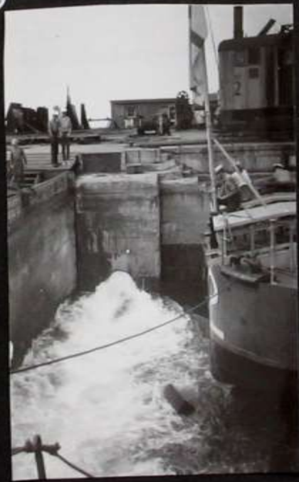
15 days later, all repairs done Flooding the dock
