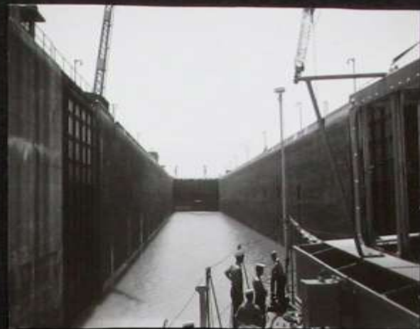
Entering the lock.
